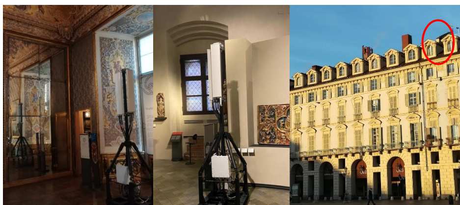
Figure 7-3: Installation for 5G indoor coverage in Sala Quattro Stagioni and Sala Acaja and rooftop antenna for the 5G outdoor coverage
